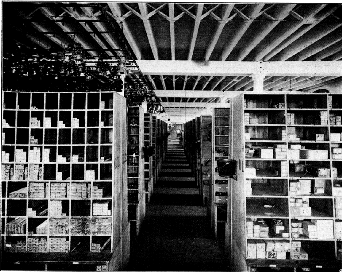
Railway Store Keepers' Association.
