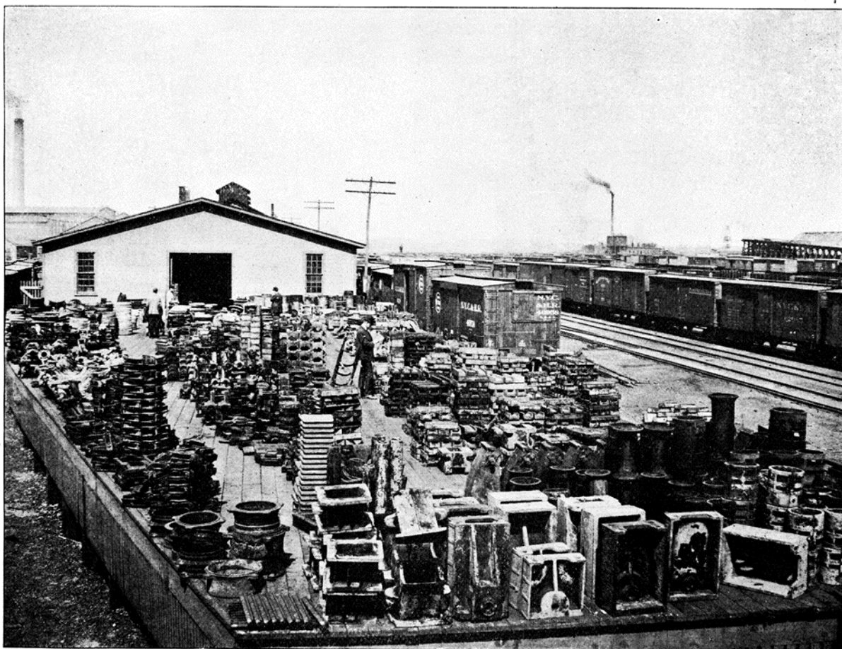
Railway Store Keepers' Association. CASTING PLATFORM OF GENERAL STOREHOUSE AT WEST ALBANY, N. Y., N. Y. C. & H. R. R. R.
