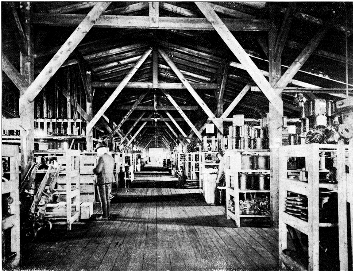
Railway Store Keepers' Association. METHOD OF STORING MATERIAL AND SUPPLIES FOR LOCOMOTIVES IN GENERAL STOREHOUSE AT WEST ALBANY, N. Y., N. Y. C. & H. R. R. R.
