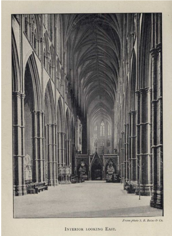
INTERIOR LOOKING EAST.
